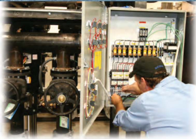
Wiring a Class "S" Deaerator
